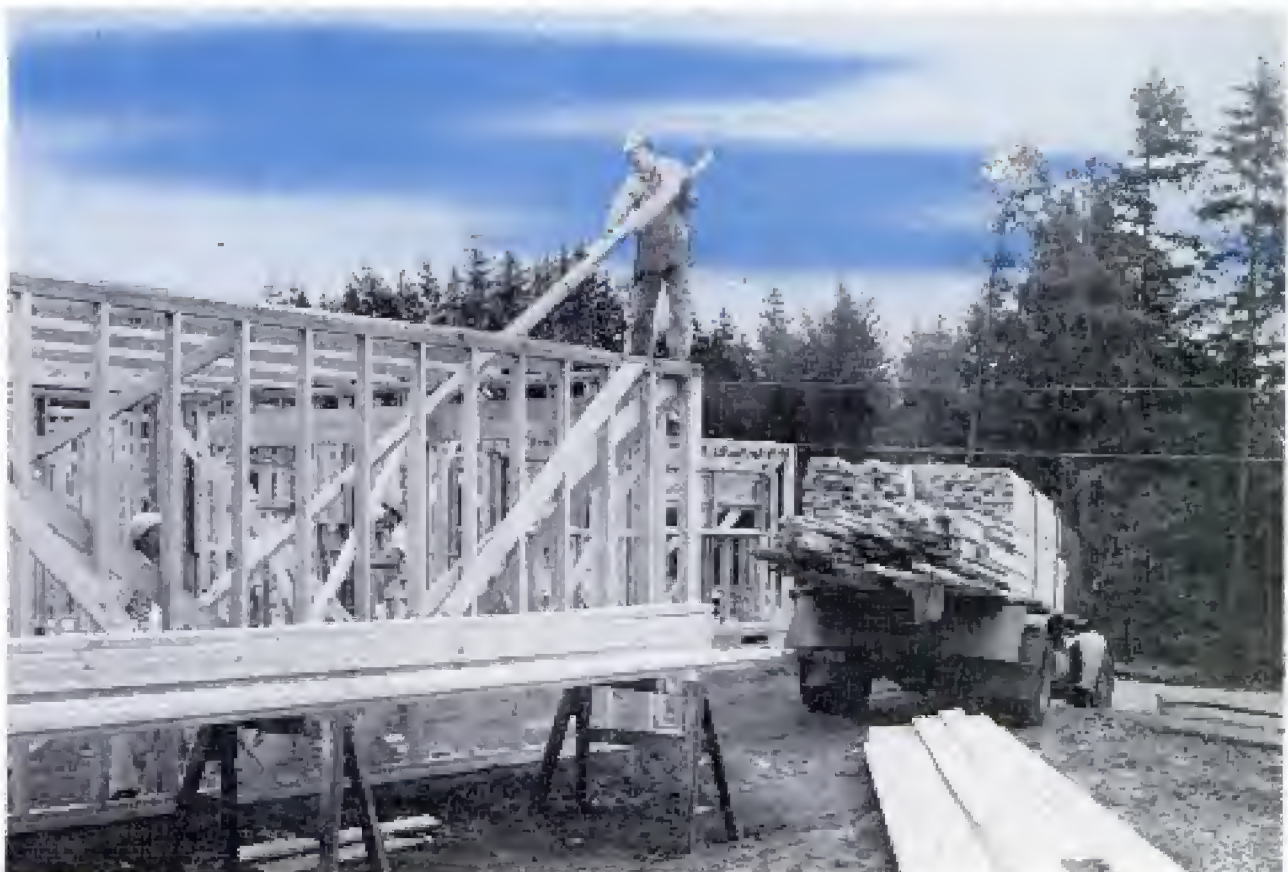
Scene of a standard-construction job—uncut lumber and other materials are delivered by local dealers
